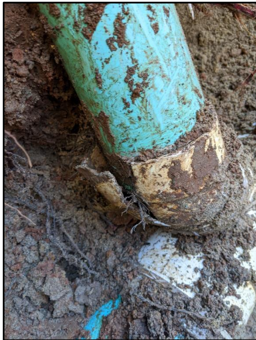
Repair Root intrusion at broken lateral fitting
