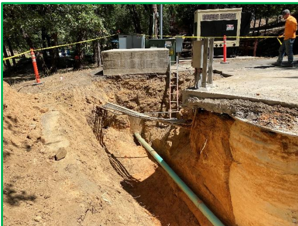
Excavating around Electrical conduits
