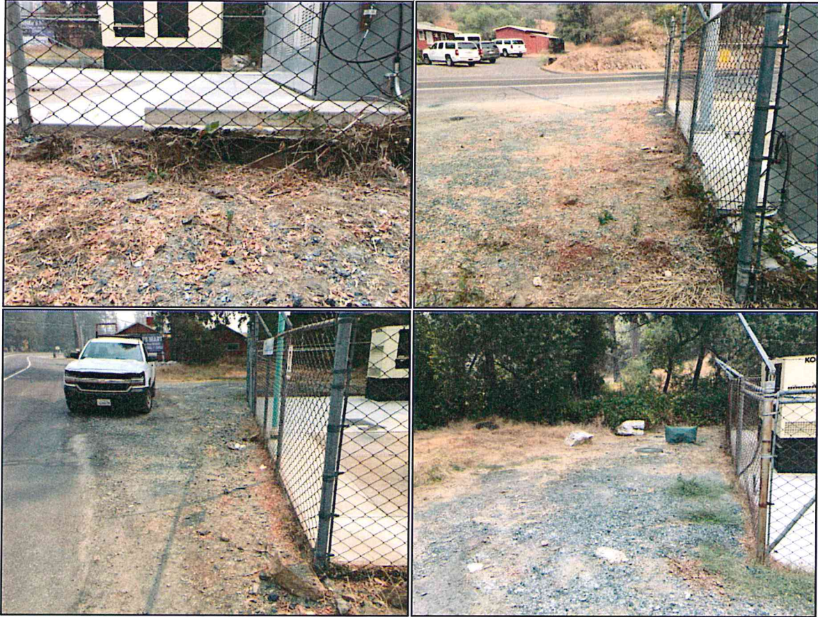
H. Lift Station 16 Parking and Road Area
