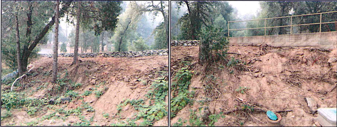
A. District Entrance Road Shoulder
