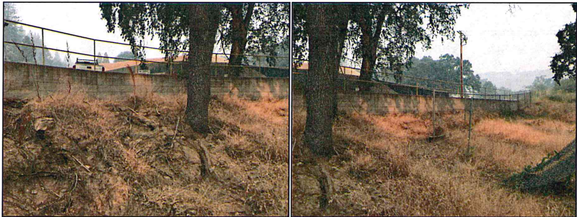
A. Concrete Footing
