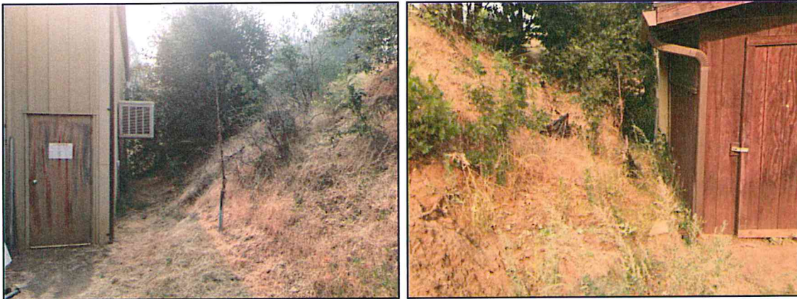
Bid Item #2 Soil Depoist Behind Maitenance Shop
