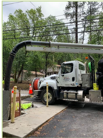
VAC-CON Vacuum Truck with boom extended cleaning LS 6
