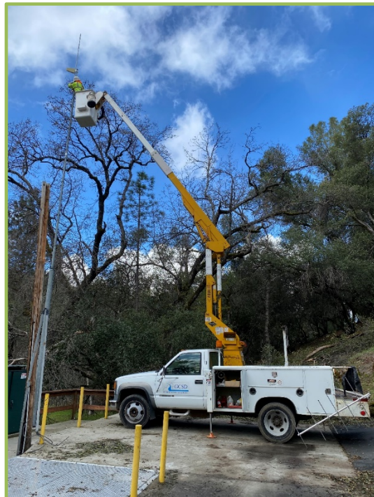
Staff Replacing Radio antenna at LS 11
