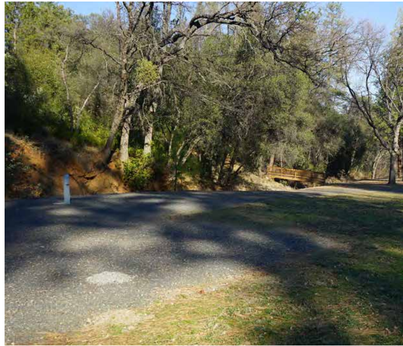
Clean up utility installations.
