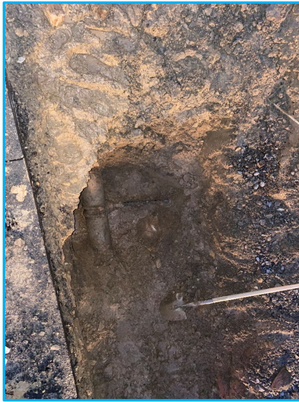
Saddle on old service failed, staff replaced with new saddle, shutoff.
