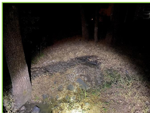
Manhole Spilling due to root blockage
